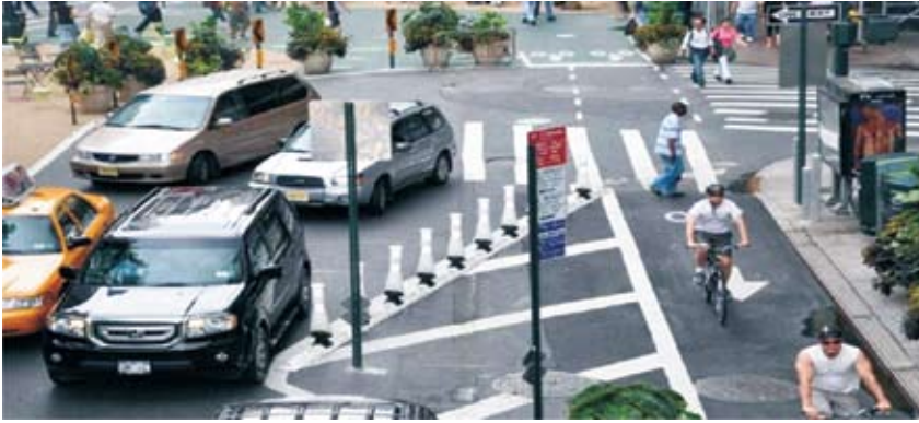
Figure 6: New York City reduced its lane widths from 3.5 m to 2.75 m to prevent speeding
