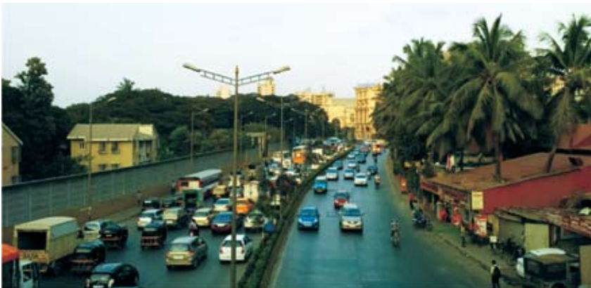
Figure 7: New roads like the JVLR in Mumbai have ignored the principles of increased capacity and equitable distribution of space
