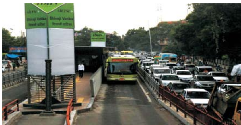
Figure 5: In Indore, the capacity of a single BRT lane is vastly more than the two lanes of general traffic
